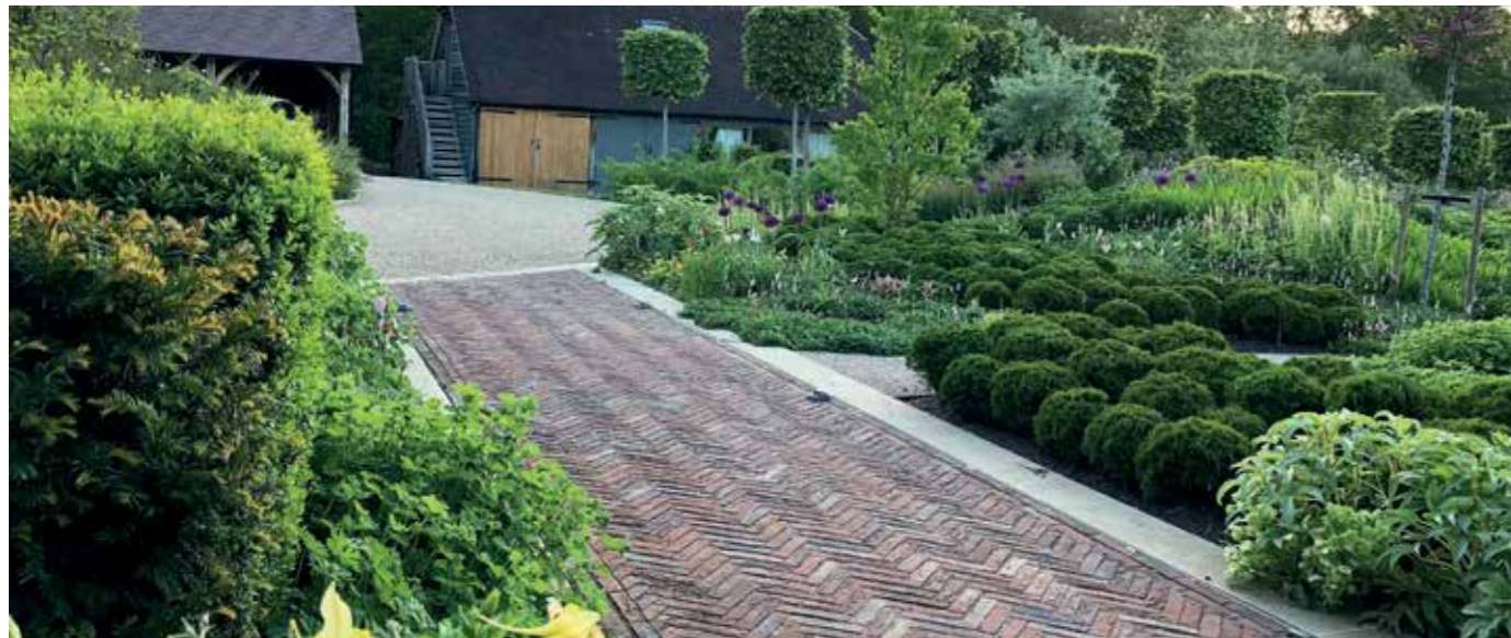
Brick path laid to camber with slot drains either side
