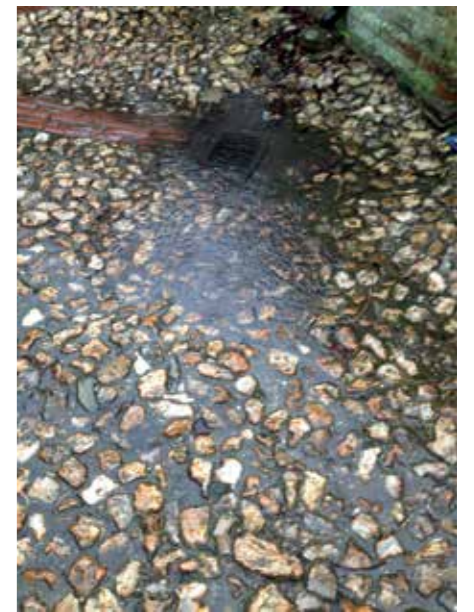
Top: Courtyard with drainage using reclaimed flint
